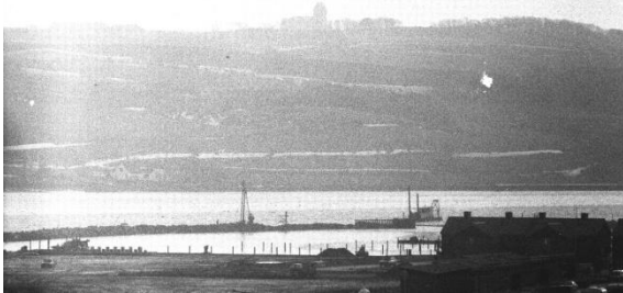
Lemvig Marina under etablering i 1976
